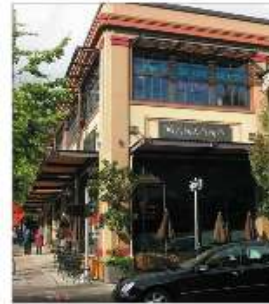
Use appropriate exterior or facade integrated (seasonal) sun shading devices at fenestration with direct solar exposures.
